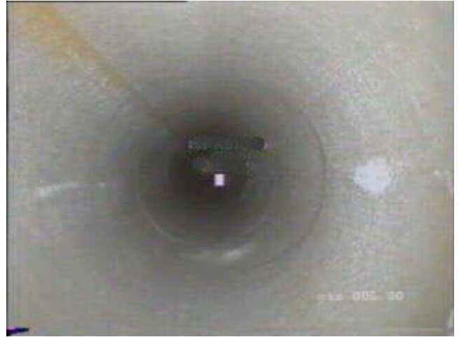
AFTER REFORMING AND RELINING
