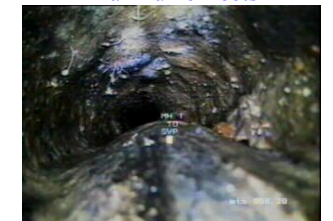
Deformed pitch fibre
