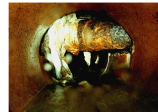
Service pipe through drain
