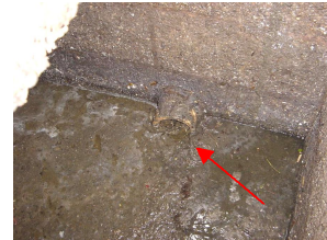
Dip-pipes missing
