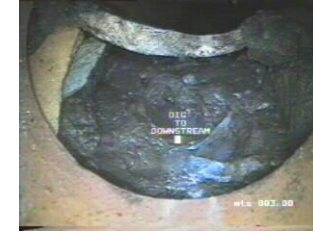
Collapsed drain
